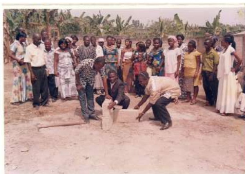
SWORD CUTTING & BRICK LAYING FOR THE CONSTRUCTION OF THE MISSION HOUSE
